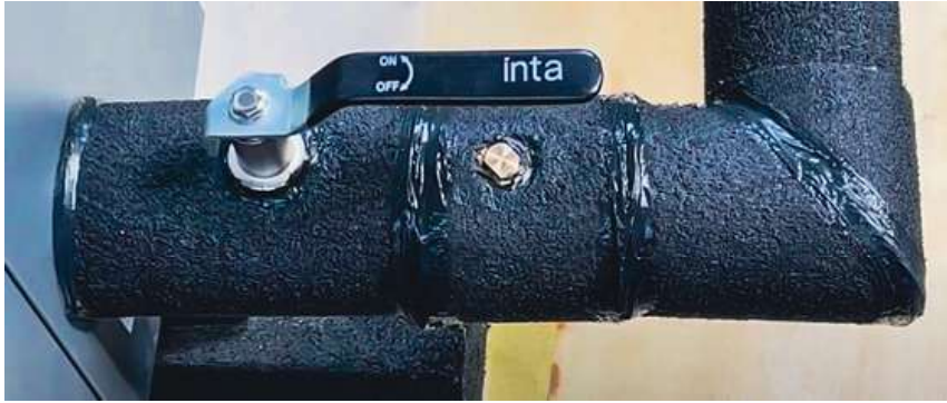
Sealing of isolation valve, antifreeze valve, 90° elbow and bonding to heat pump.
