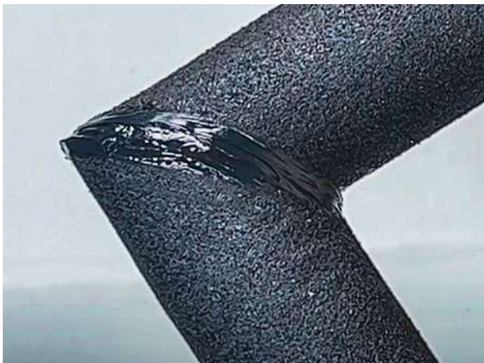
Sealing and capping to 90° elbow.
