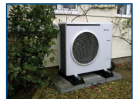
5. Secure the ASHP units onto the kit - the installation is complete.
