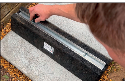
STEP 10 - Secure the feet with the nuts and washers, and position the spring nuts in the strut.
