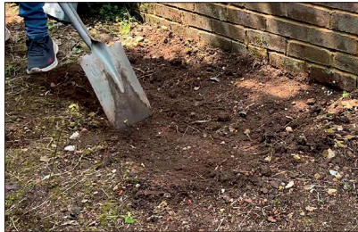
STEP 2 - Prepare the ground.
