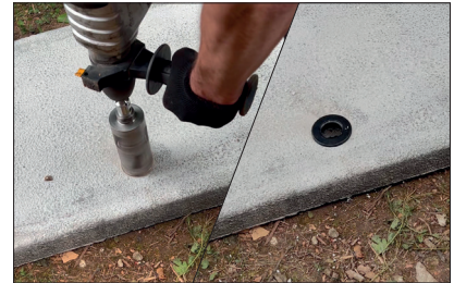
STEP 3 - Drill the slab for insertion of pipework and insert the drainage bung.
