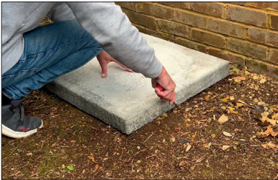
STEP 1 - Position and mark ground for the required location of the FLEXI Lite Slab.
