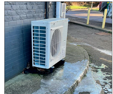
USING THE SOAK-AWAY PREVENTS THE CONDENSATE FROM FLOWING ONTO PATHS AND FREEZING - CAUSING A SLIP HAZARD.
