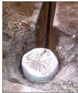
SHOWING THE INSTALLATION BELOW GROUND OF THE ASHP SOAK-AWAY.
