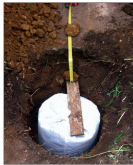
SHOWING THE INSTALLATION BELOW GROUND OF THE ASHP SOAK-AWAY.
